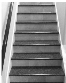
g Indoor marble stairs
