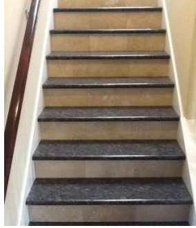
a Indoor marble stairs
